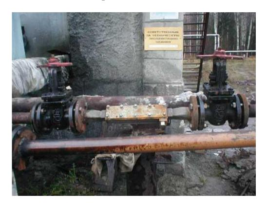
Dispersers with 3-24 tons per hour capacity.
