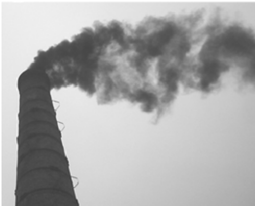
Boiler-house exhaust on regular mazut (low grade heating oil)
