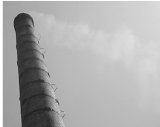
Same boiler-house exhaust on water/mazut (low grade heating oil) mixture after emulsion processing
